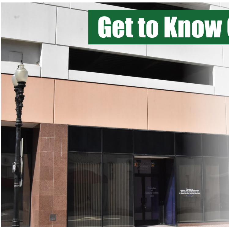
Custodian of Records Office, 200 W. Santa Ana Blvd., Santa Ana. Entrance on Sycamore Street near 5th Street.
