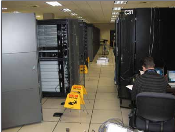
HCA servers installed in racks at the OC Data Center.
