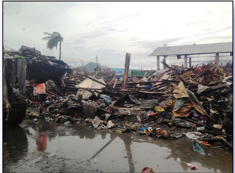
Typhoon Haiyan, with winds at 160 to 195 miles per hour and a storm surge of up to 20 feet, overwhelmed provinces within the Philippines. Approximately 500,000 homes remain destroyed.
