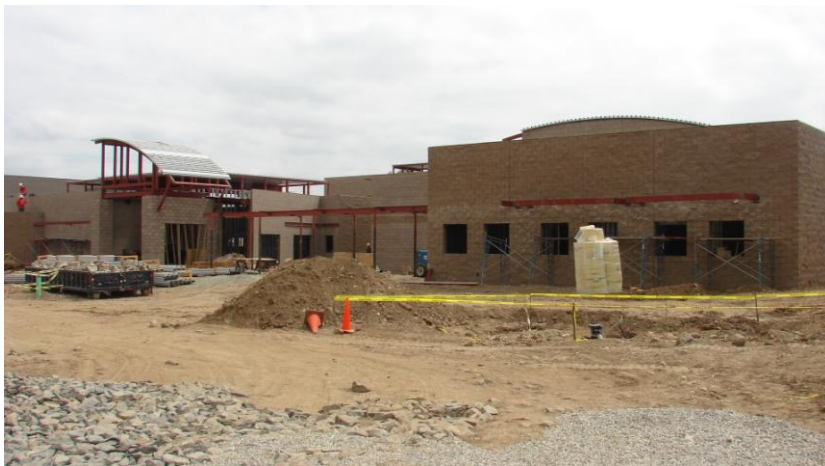
Construction Progress July 2011
