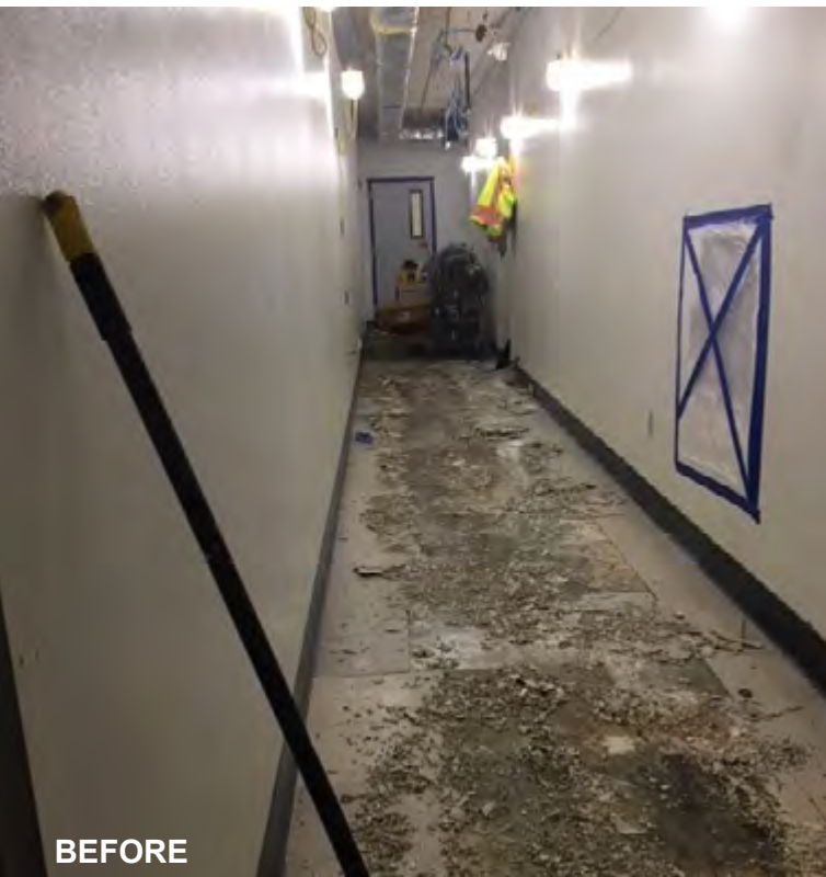
Demolition of flooring in a common hallway (phase 2).
