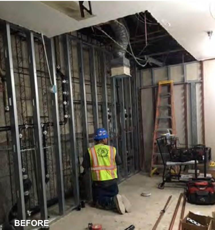
Construction workers install plumbing for new restroom fixtures in the men's employee restroom (phase 1).
